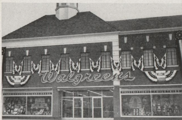
HAMPTON VILLAGE, St. Louis —An utterly different Walgreen Store in the world's largest drive-in shopping center. Massive-sized departments, plus a most modern Prescription Laboratory, made it the talk of St. Louis.
